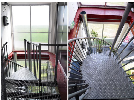
Indoor stair handrail
